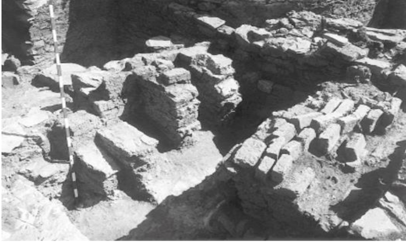
Fig. 7 Kiln Structures in the Small Bath in Anemurium (Keser, 2019: 195 Res. 40)
